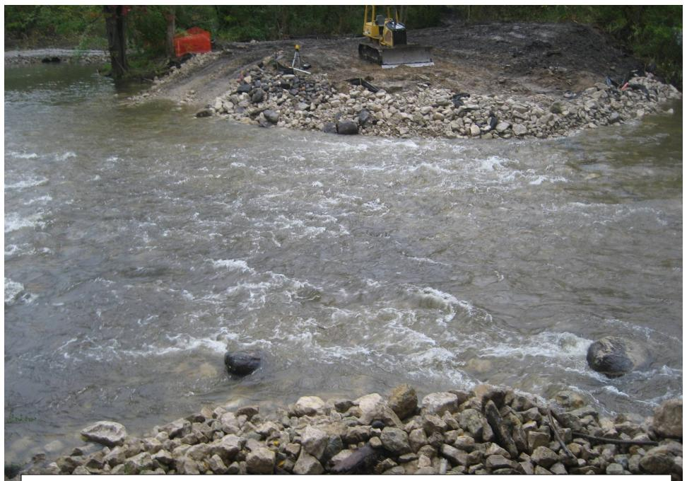
Spillway dam restoration, riffle installation and rough grading complete - 9/30/11
