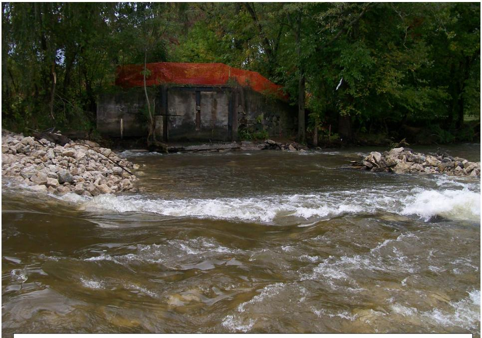
Spillway dam removal, west half complete and east half of dike breached - 9/28/11
