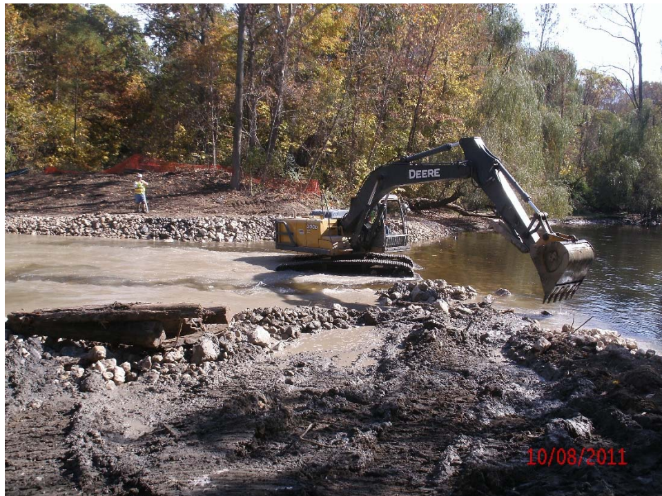
Diversion dam riffle installation - 10/8/11.
