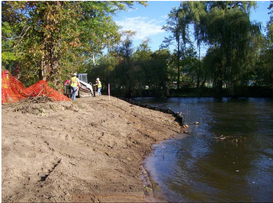
Spillway dam start of streambank grading and stabilization.
