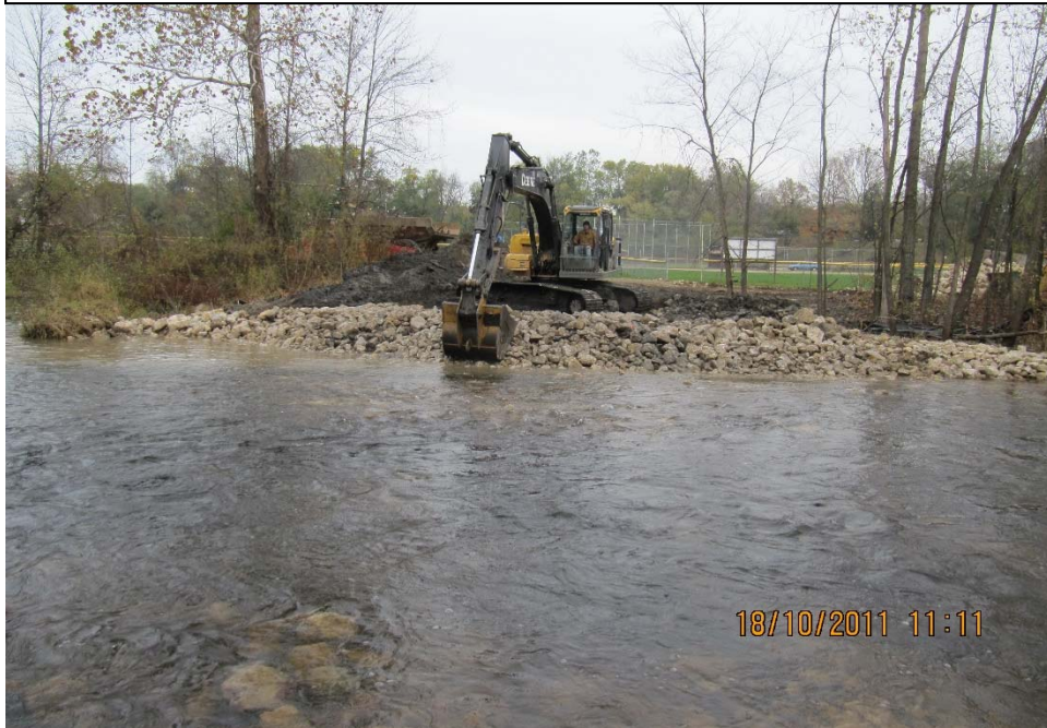
Start of historic channel bankfull bench and riffle construction - 10/18/11.
