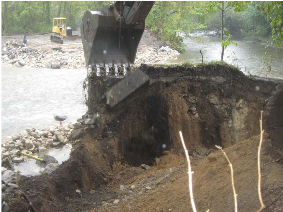
Removal of east wingwalls and abutment at spillway dam.
