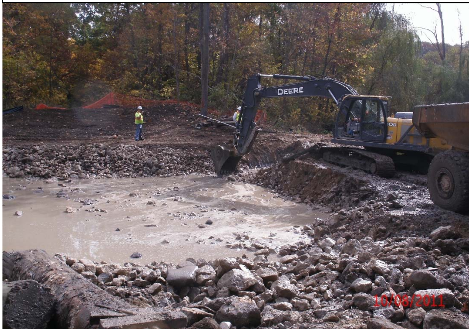
Start of diversion dam cofferdam breach - 10/8/11.
