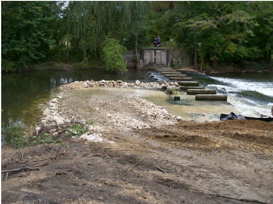
Installation of upstream and downstream rock cofferdams at spillway dam.
