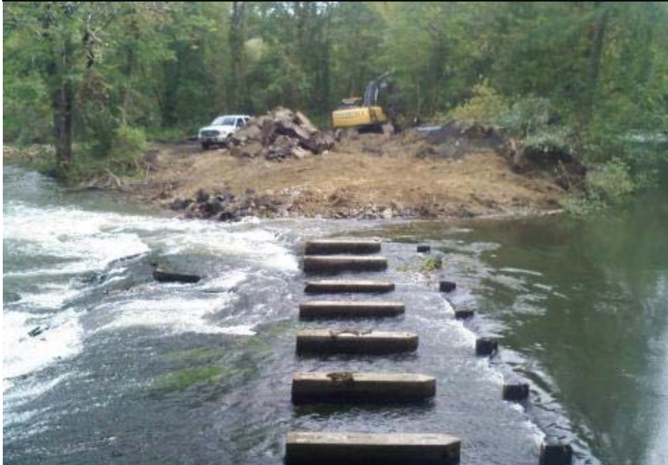
Start of spillway dam east wingwall and abutment demolition.
