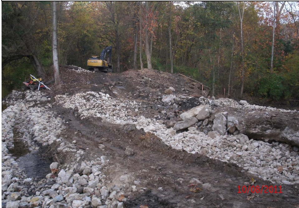
Diversion dam upstream rock cofferdam installation - 10/8/11.
