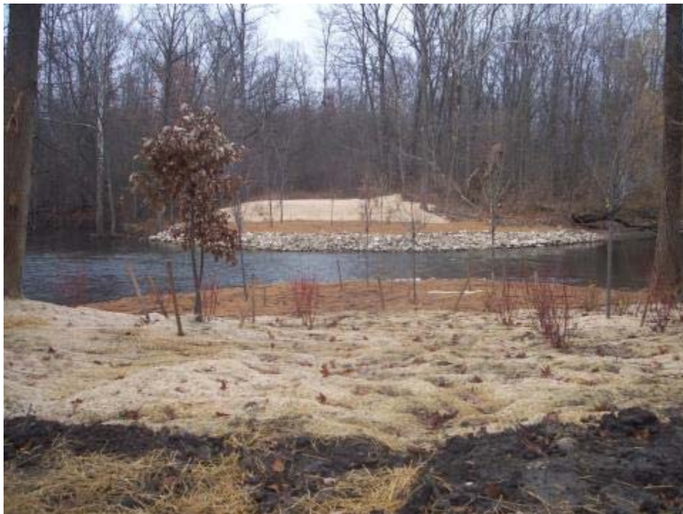
Figure 6-2. Diversion dam (center) constructed riffle and bankfull benches after dam removal.
