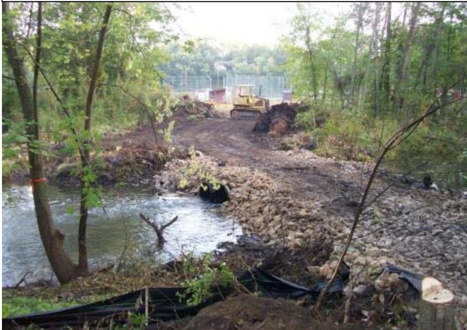
Historic channel crossing preparation - culvert installation.
