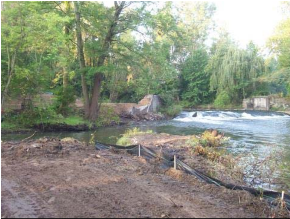
Start of spillway dam east wingwall and abutment demolition.
