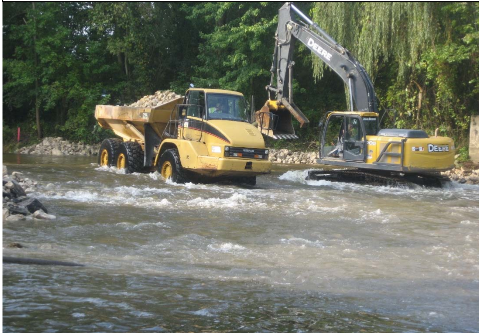
Installation of spillway dam riffle.
