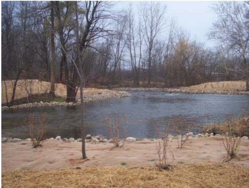
Figure 6-1. Historic channel (left) and spillway dam (center) constructed riffles and bankfull benches after dam removal.
