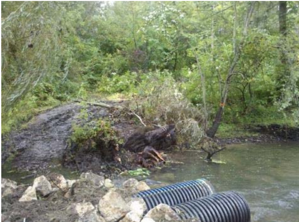
Historic channel crossing preparation - culvert installation.
