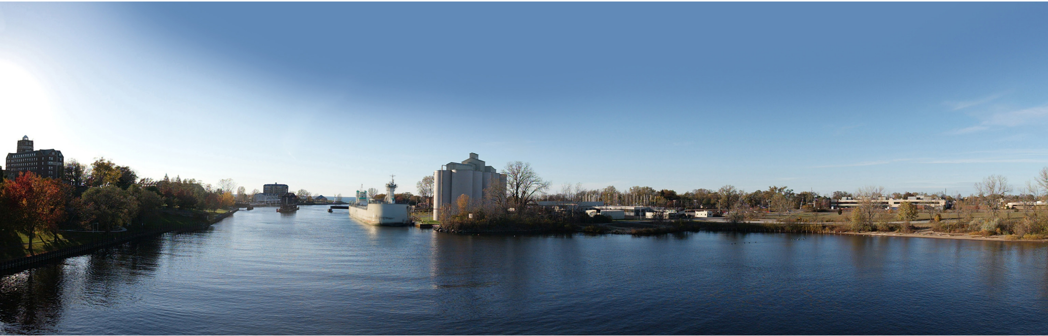
Existing View of Outer Harbor from M.63 Blossomland Bridge Refer to pages 4, 5, 24 and 30
