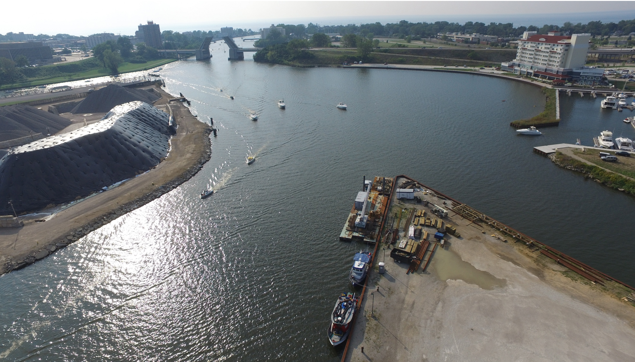
Existing View of Twin Cities Harbor looking West Refer to pages 16 and 55
