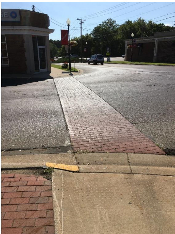
Figure 7: Faded Crosswalk Marking
