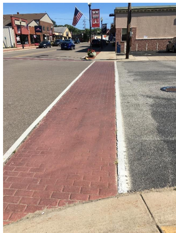
Figure 8: Crosswalk Marking in Good Condition
