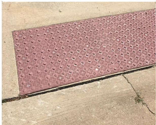
Figure 6: Detectable Warning in Good Condition
