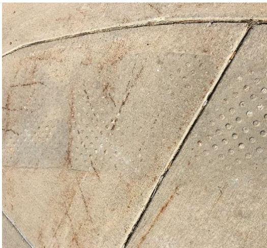
Figure 5: Detectable Warning in Fair/Poor Condition
