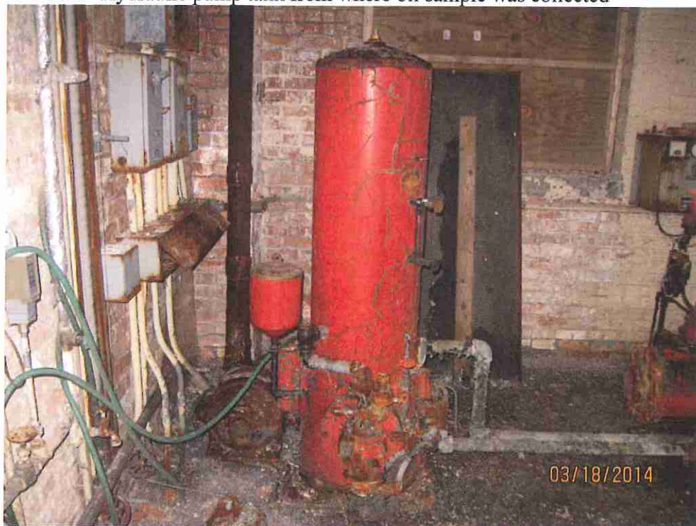
Hydraulic pump tank from where oil sample was collected
