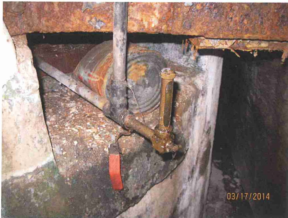
Petcock valve on side of generator where oil sample was collected
