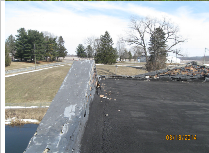
Asbestos containing roofing tar (HM-12) covering the generator room roof.
