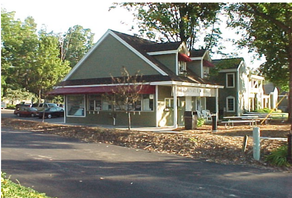
Eventual development of a small-scale commercial node is anticipated in the Township
