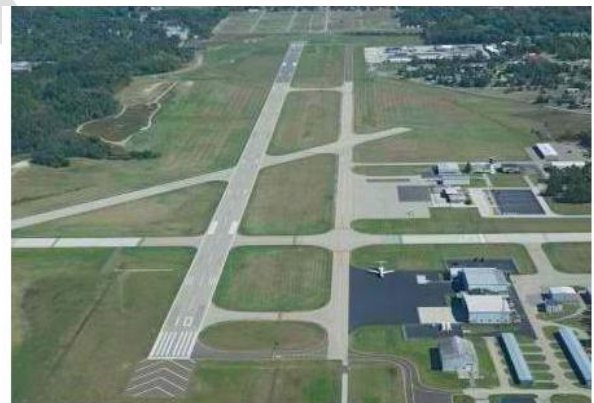
Southwest Michigan Regional Airport
