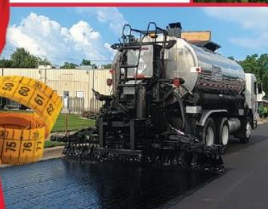
Emulsion being applied to scratch course prior to GlassPav 50 installation.
