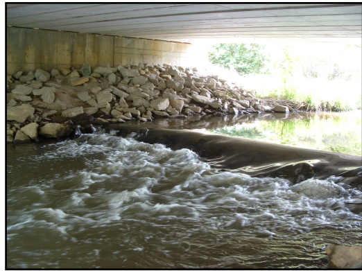
Figure 1: Head loss at M-63/Niles Ave
