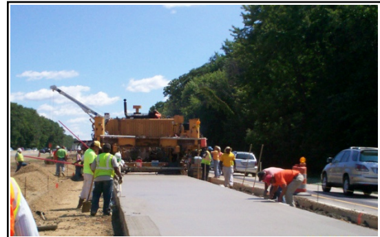
MDOT working to rebuild trunkline roadways.
