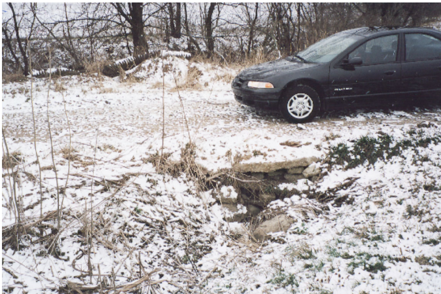
Photograph 11: Blocked Driveway Culvert
