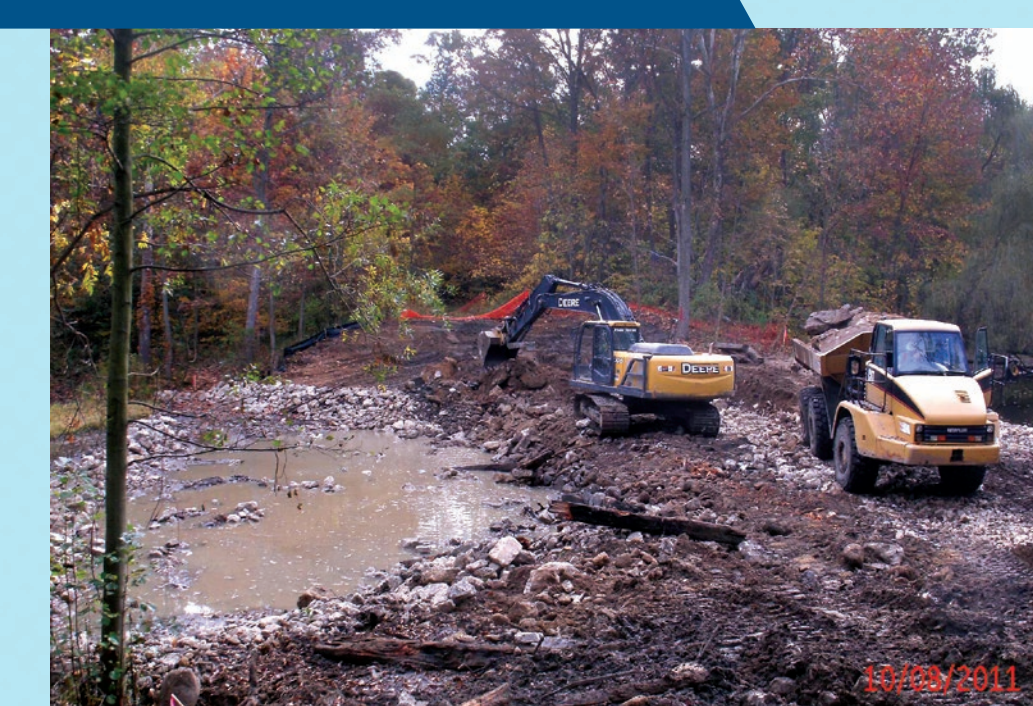
Diversion Dam removal
