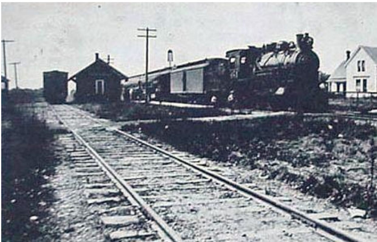
An old view of the depot at Stevensville, MI with a Pere Marquette passenger train taking on passengers ( michiganrailroads.com .)
