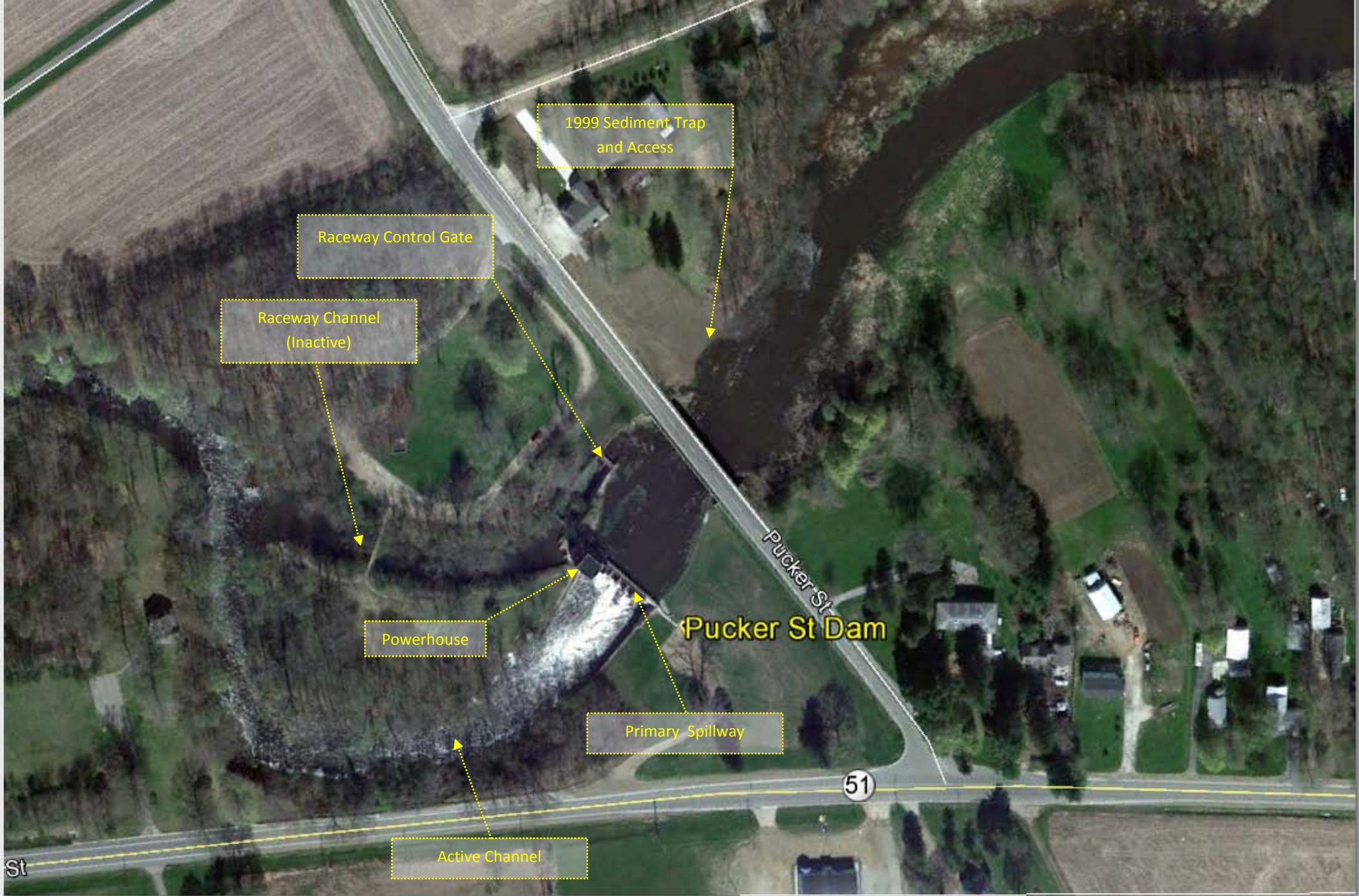
Figure 5: Salient features near and around the dam.
