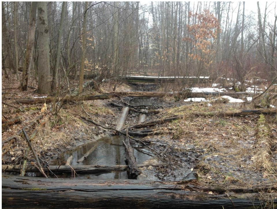
Figure 50. The old crossing above the pond - note the two old pipes in the bed
