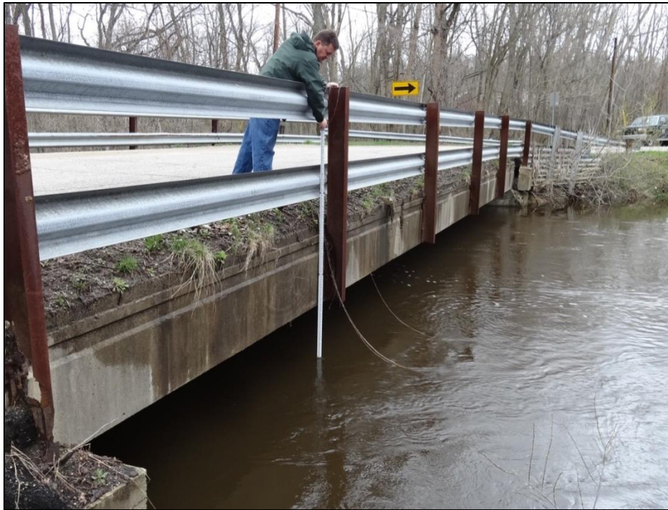
Figure 60. Example of how water surface elevations were measured with reference to the low chords of the bridges during the April, 2013 flood. This is at Sink Rd. (photo provided by Robert Frank).
