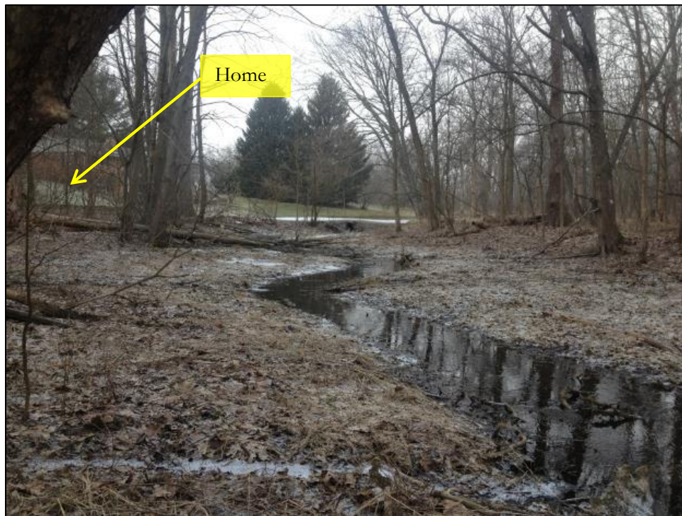
Figure 62. Photo (looking upstream) of the relict channel that may be re-occupied near the home approximately 1,000 feet upstream of Sink Rd. on the west side of the valley.
