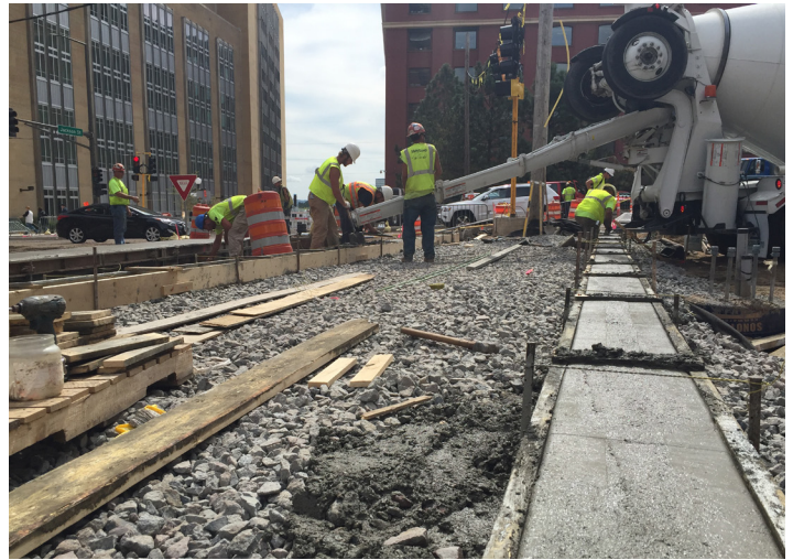
Construction on Jackson Street in Saint Paul, MN
