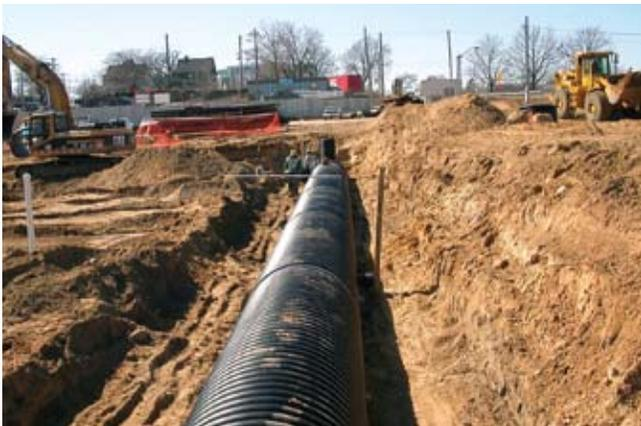
*Subsurface infiltration system*
