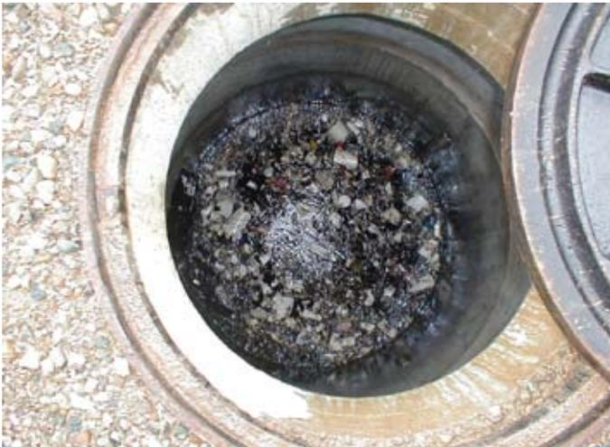
*Screening vortex device with floating debris*
