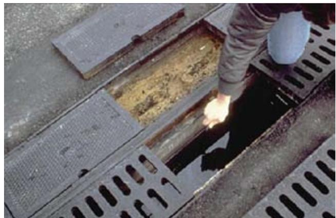
*Linear perimeter filter in trench drain*
