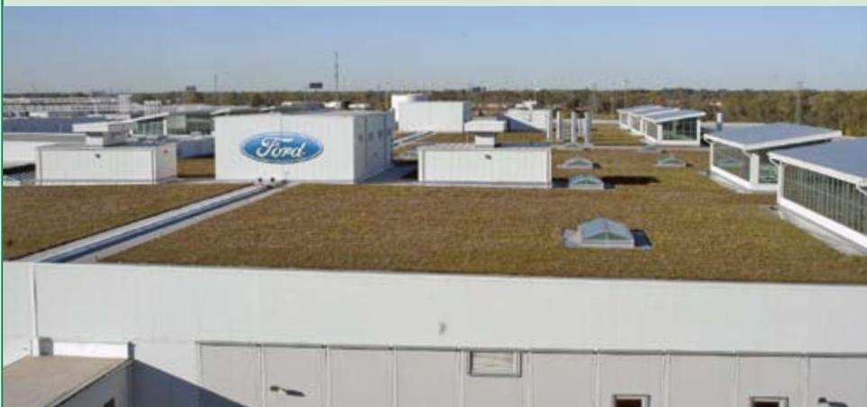
*Recognized in 2004 by Guinness World Records as the largest green roof in the world, this green roof covers 454,000 square feet atop Ford's truck assembly plant in Dearborn, MI. The green roof is part of a comprehensive effort to revitalize the historic Ford Rouge complex as a model for 21st Century sustainable manufacturing and is a significant component of a site-wide 600-acre stormwater management system.*
