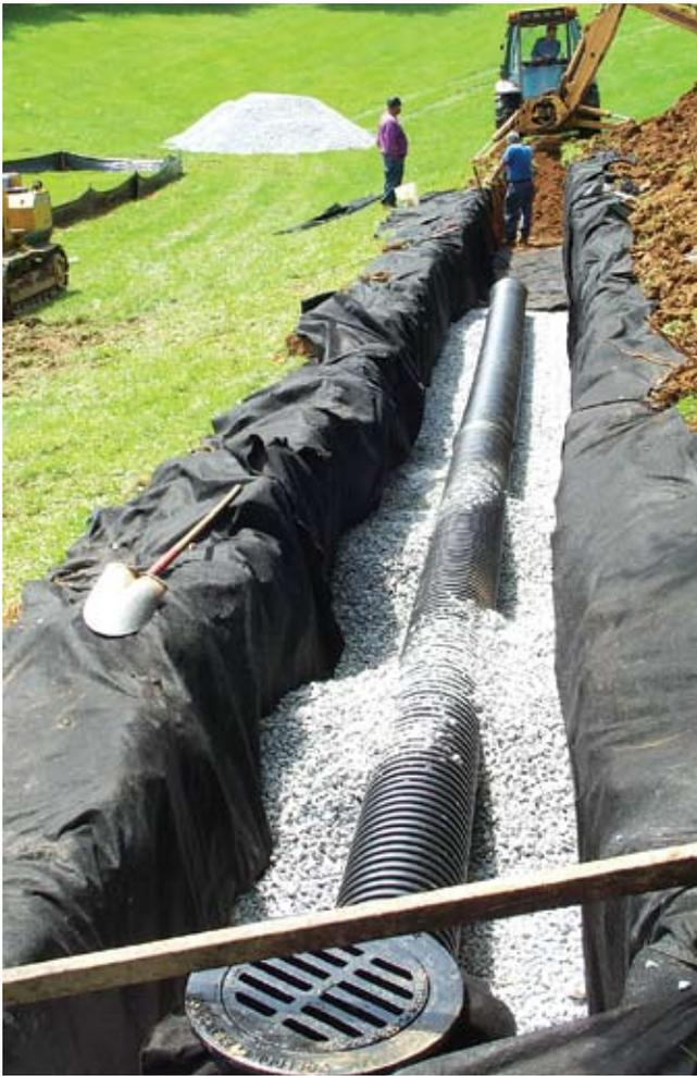
*Infiltration trench with geotextile*
