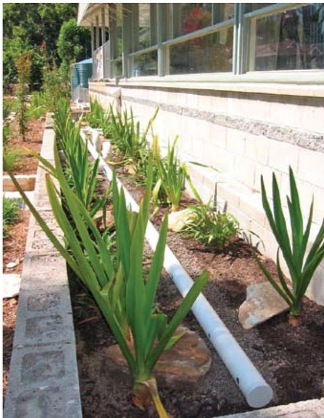
*Perforated pipe used for inflow/distribution in a stormwater planter box*
