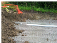
Gravel Base and Underdrain
