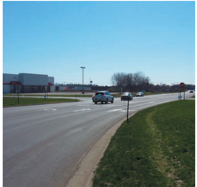
Image of Mall Drive between a set of large apartment complexes and retail centers containing several bus stops; road showing five traffic lanes without sidewalks, bike lanes/shoulders, or intersection crossings; grass showing signs of heavy pedestrian use
