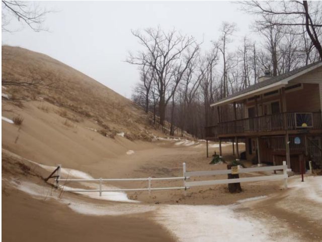
This picture was taken in early 2012. Dune has migrated closer to this home along the County owned dune property.
