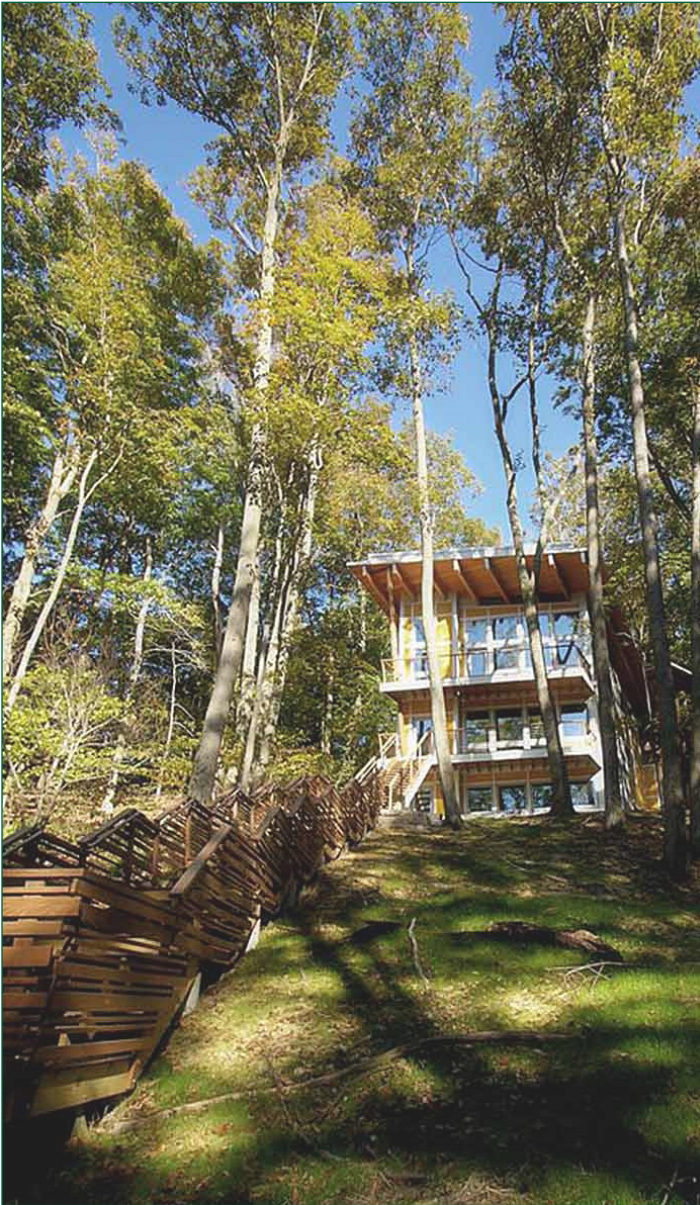
House from parking area - steps to left
