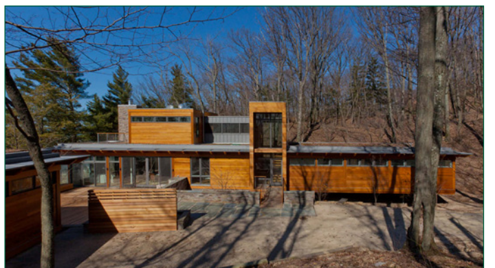
Green roof used to moderate heating and cooling, and extend life of roofing. [18]
