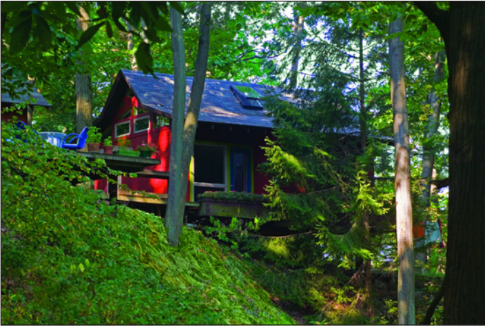
Modular approach used on site with small area of level land. [6]
