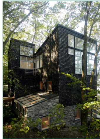
View from North
