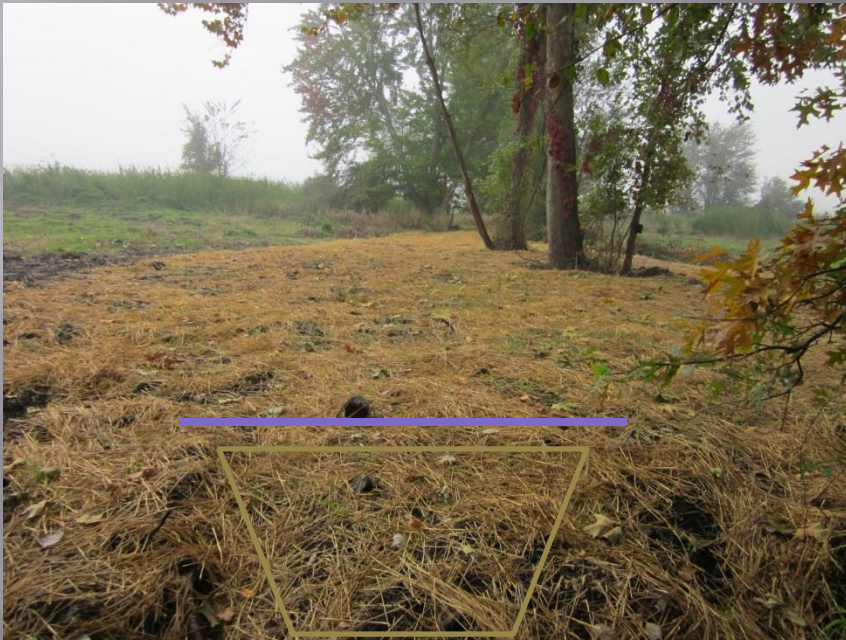
Surface ditch plugged during restoration
