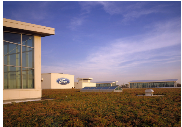
Expansive green roof on the Ford Rouge Plant in Dearborn, Michigan. www.thehenryford.org/rouge/livingroof.asp
