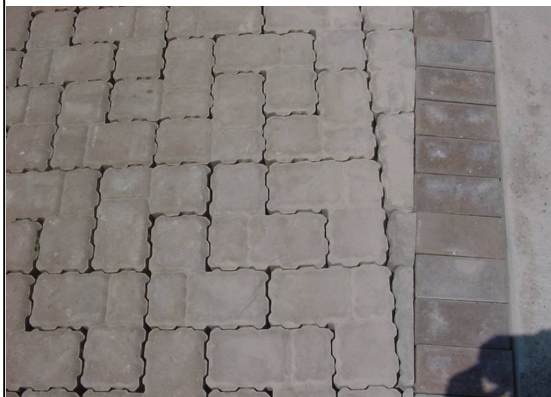
Porous pavers in the Pokagon Development.
