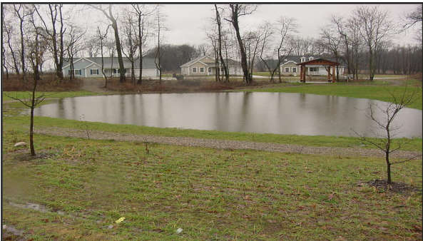
One feature within the development is large lowland areas that naturally fill with stormwater. These pools allow natural groundwater recharge to occur.
