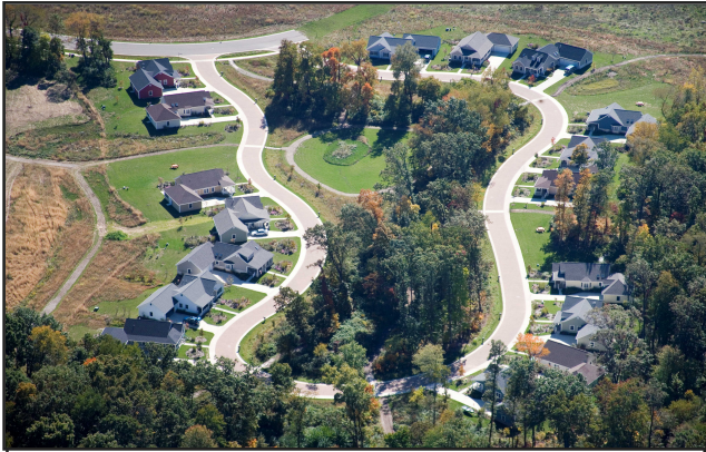
The photograph above highlights narrowed road widths, permeable roadways, vegetated storm swales and preserved open space.
