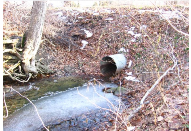
Site Q Before: The road bank was eroding under and behind the culvert outlet, impairing water quality by adding soil sediment.
