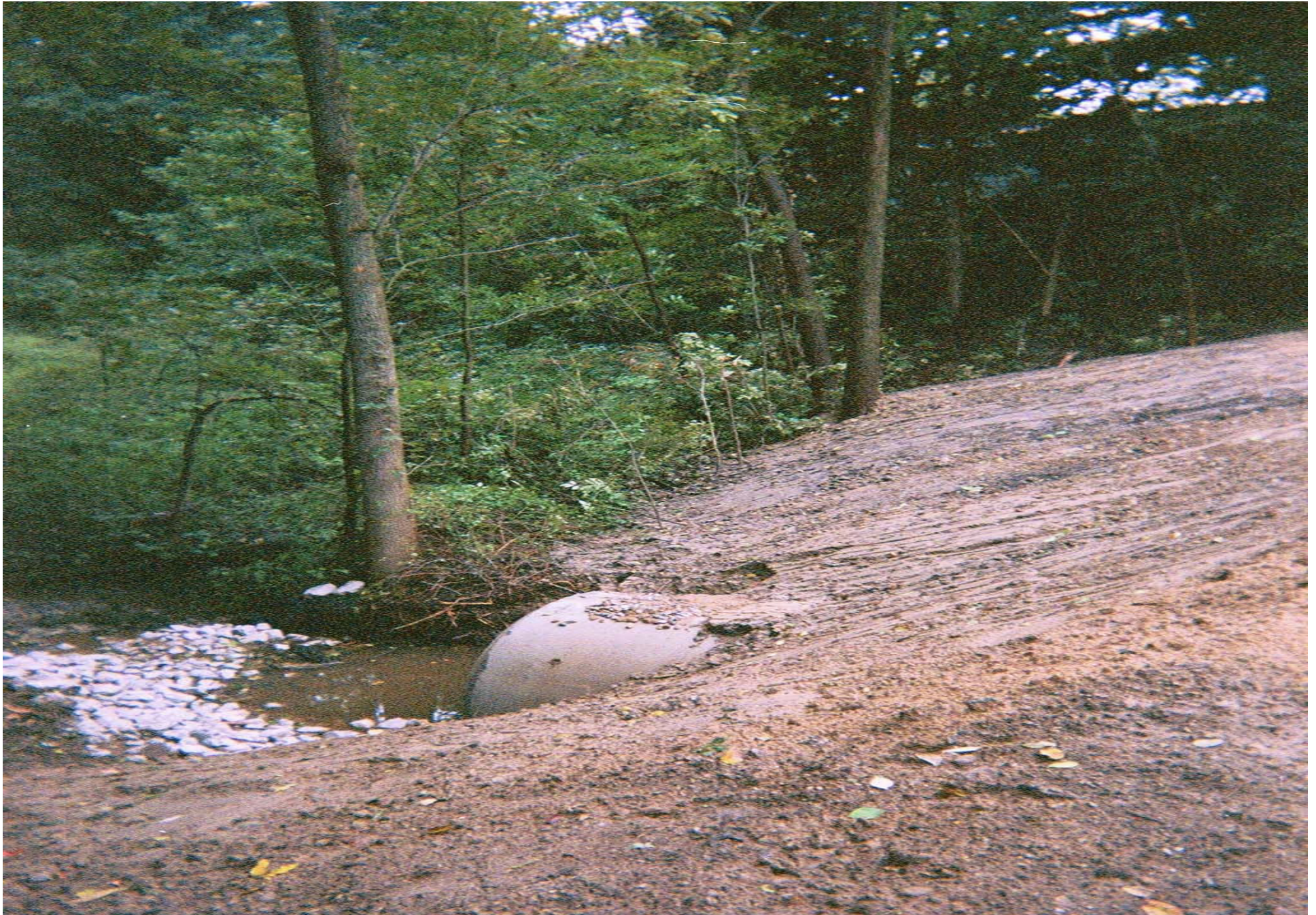
Lack of Sufficient Buffer/Filter Strip
