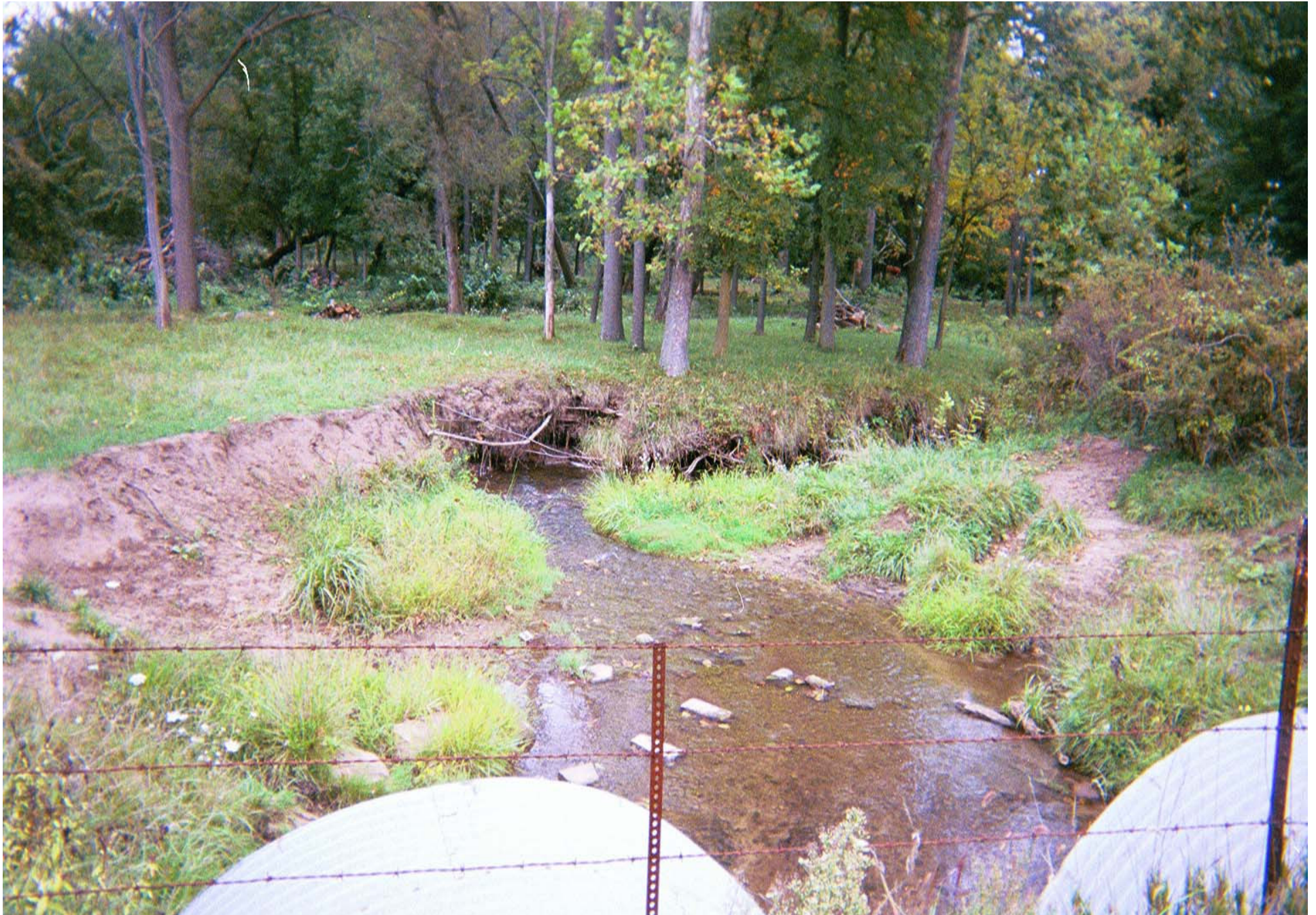
Lack of Stabilized Outlets
