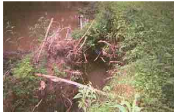
Photograph 2: Erosion from Diverted Flow at Root Mass
