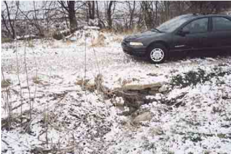
Photograph 11: Blocked Driveway Culvert
