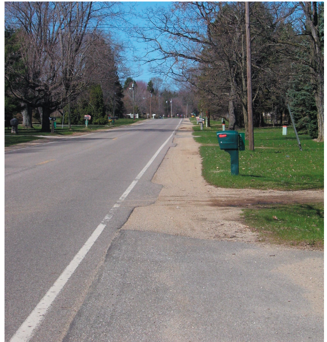
Wide, unpaved should on north side of Pipestone Rd., between Nickerson Rd. and River Rd.
