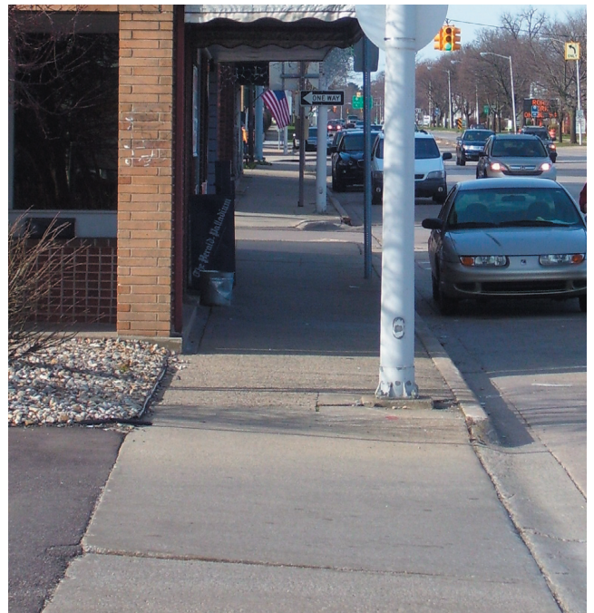
Obstacles in sidewalk and rough grading on east side of Main St., between Ship and Pleasant
