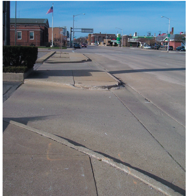
Absent curb cuts and lack of street buffers on east side of Main St., between Port St. and Ship St.
