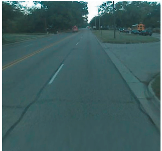
Street view of Pipestone Rd., between M-139 and Napier Ave., showing four travel lanes with no space for a shoulder or full bike lanes (photo from Google Maps)
